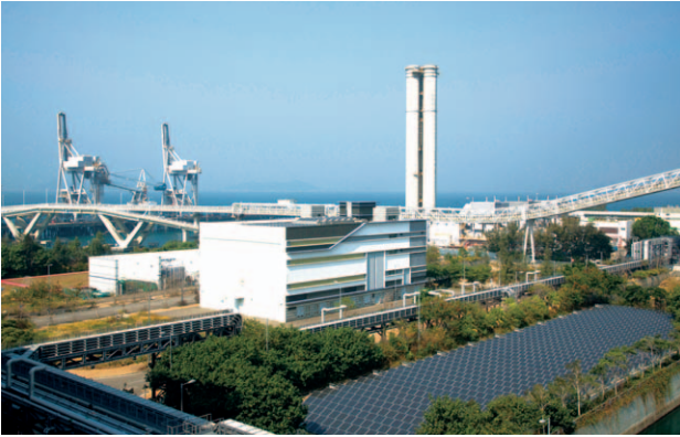
Our solar power system at LPS generated over 1 million units of electricity during the year.
