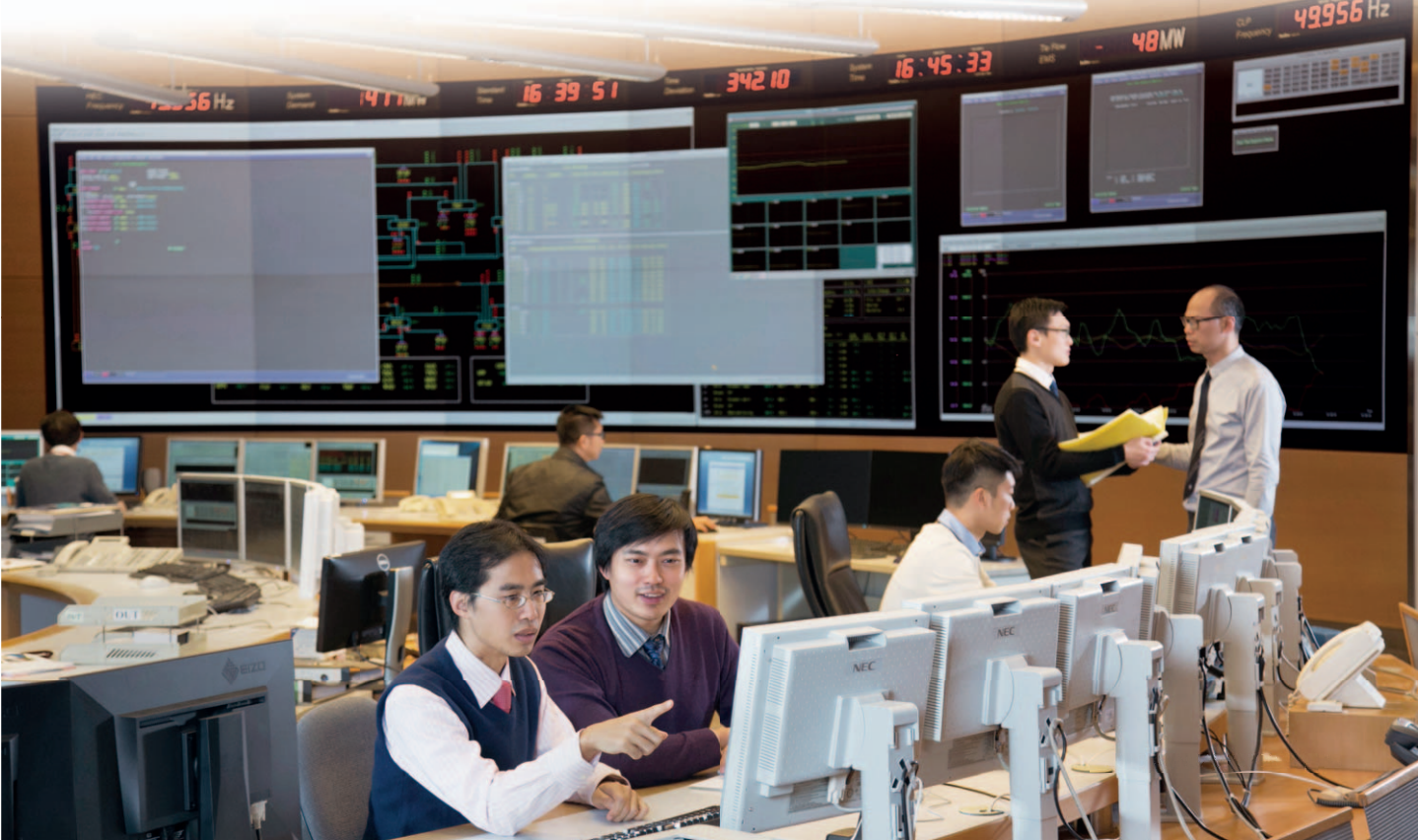
The System Control Centre runs on advanced IT platforms.
